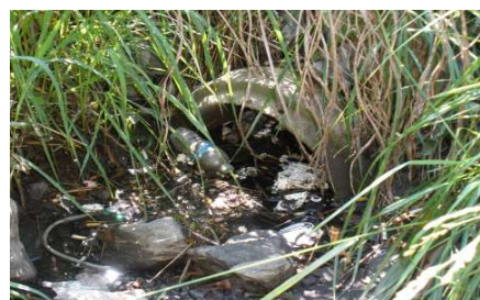
Examples: Crossline Pipes Blocked
