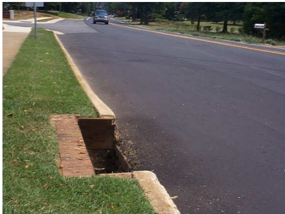
Examples: Inlets Damaged / Missing
