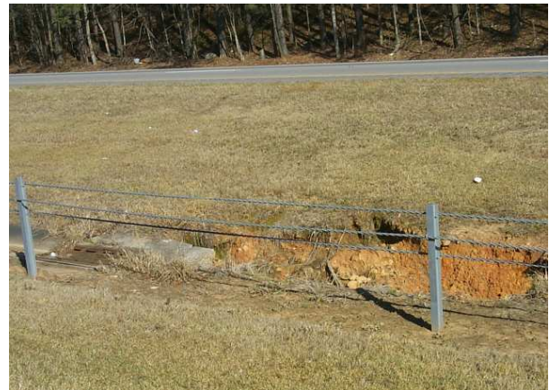
Examples: Inlets Damaged / Missing
