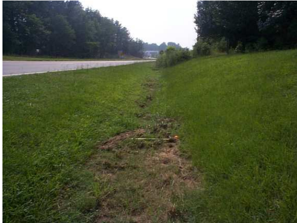
Examples: Lateral Ditches — Blocked
