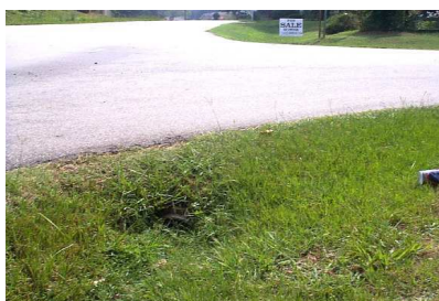
Examples: Crossline Pipes Blocked
