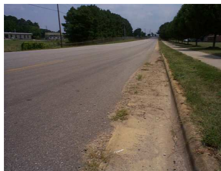
Examples: Gutters Blocked
