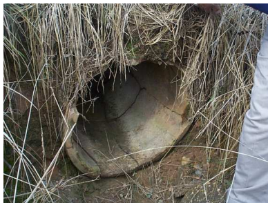
Example: Crossline Pipe Damaged
