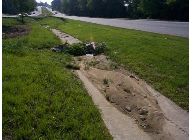
Examples: Lateral Ditches — Blocked
